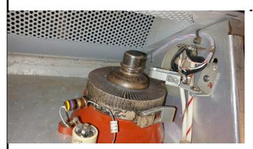
The tube compartment with tube (4CX1000A) installed and air flow detector (which was checked out with a heat gun) on discharge of tube.
